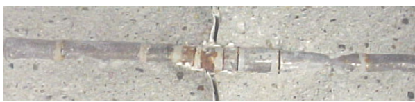
Fig. 6 Corroded steel at joint and its surroundings.
