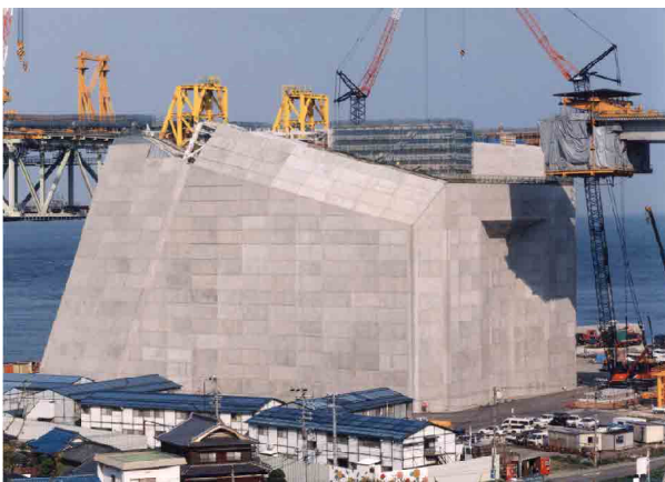
Fig. 31 Anchorage 4A of Akashi-Kaikyo bridge.
