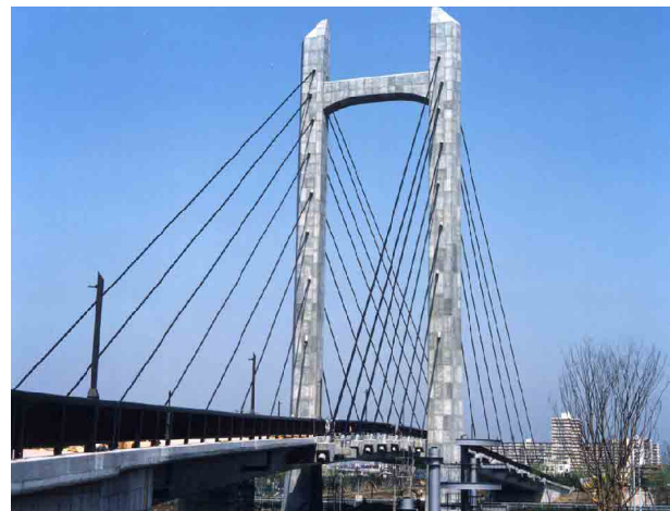
Fig. 29 Shin-kiba Ohashi bridge.
