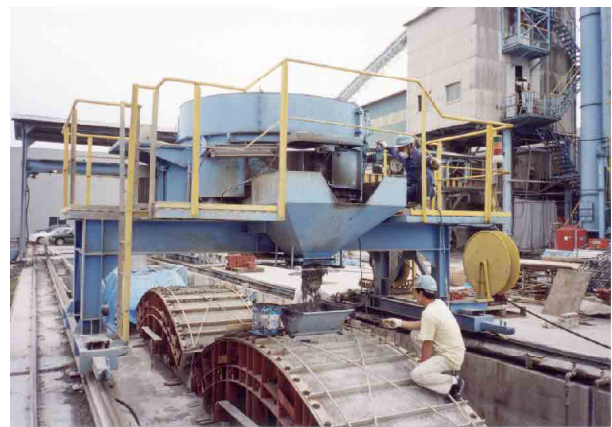
Fig. 32 Casting of SCC for Tunnel Segment.
