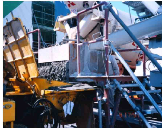
Fig. 25 Automatic acceptance test at job site.
