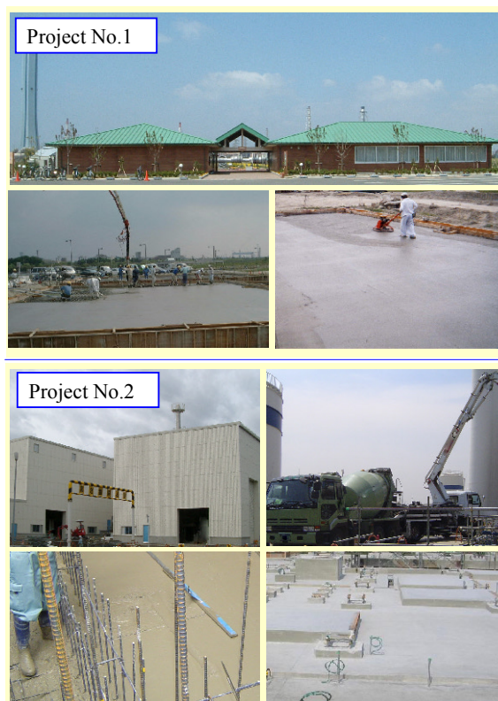
Fig. 3 Example of application to actual buildings.
